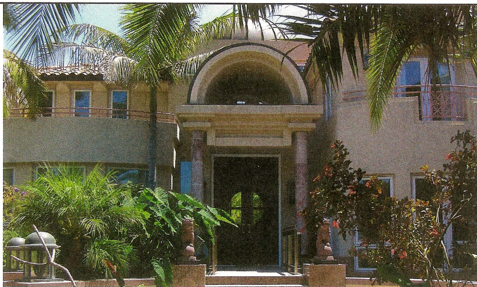
Mr. Wheeler's first construction project with steel framing is this 7,200 square foot home in Pelican Hill, Calif.
